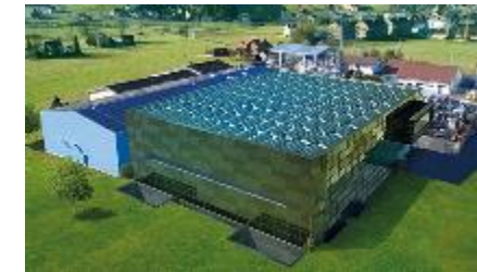
Storage of Data in Tier IV Data Center in Switzerland
